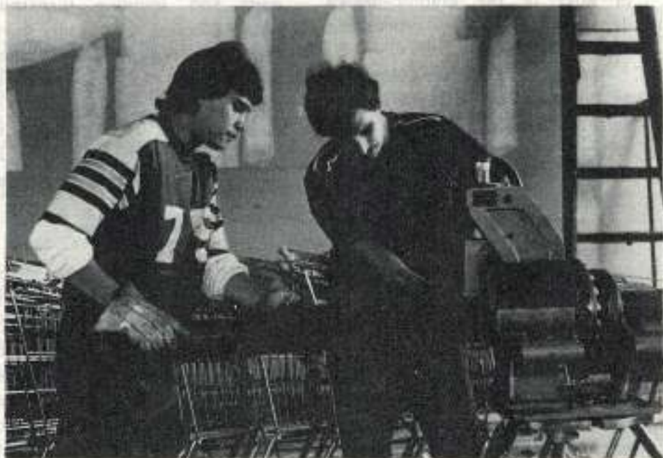
Above: Daiva Kryzanasuskas and Mary Lou Morgan in courtyard of Carrot Common. Below: Plumbers at work.
