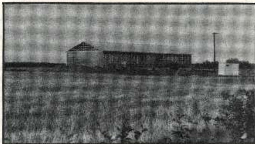
P.E.I. Potato Chip Co-operative plant under construction. Usine de la Coopérative de croustille en l'I-P.E.
